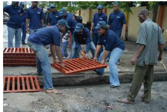
Access Bank staff Rehabilitating Public Drain Grille Cover at Karimu Kotun - Oyin Jolayemi Streets Junction, Lagos
